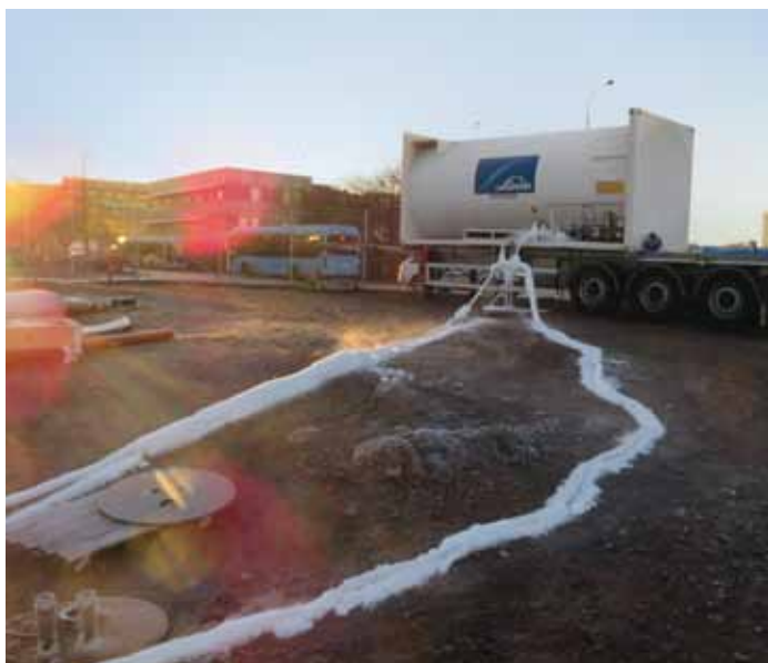
Tank and supply lines for freezing project
