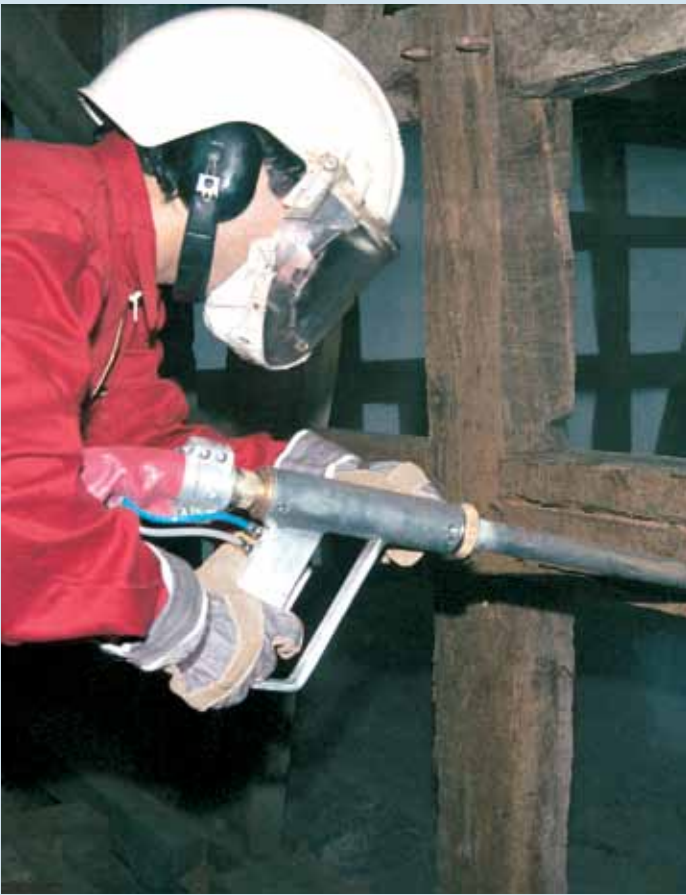
When dry ice blasting (e.g. when renovating an old half-timbered house, as shown here), always wear protective clothing.
