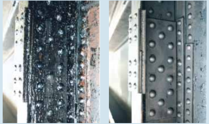
Removing resinated oil for renovation purposes.
