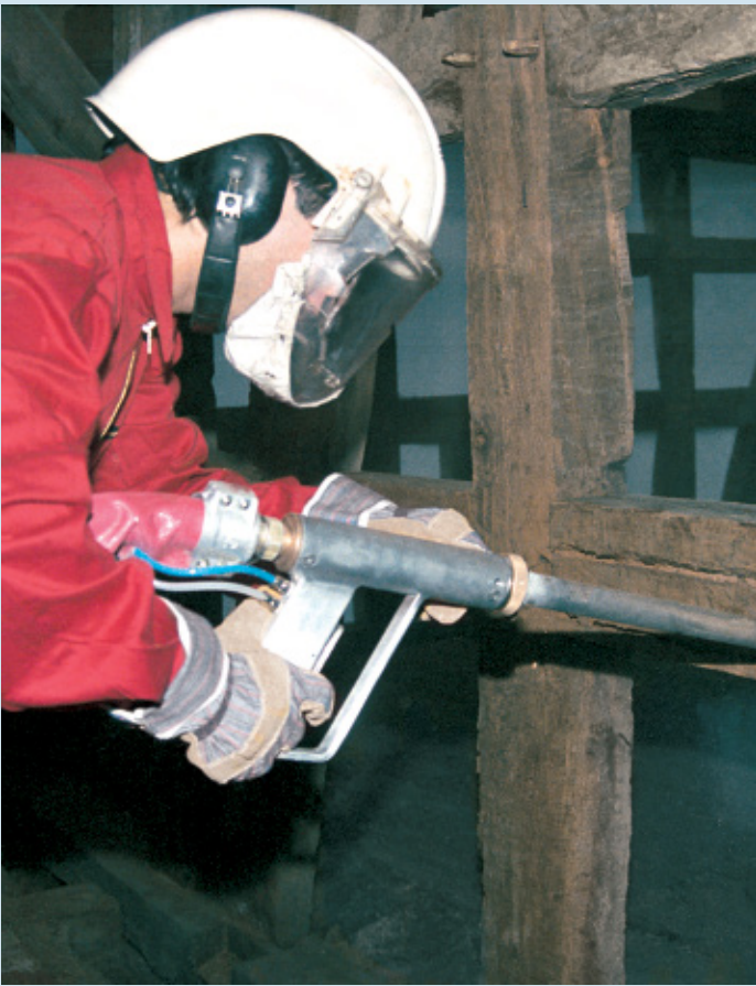
When dry ice blasting (e.g. when renovating an old half-timbered house, as shown here), always wear protective clothing.
