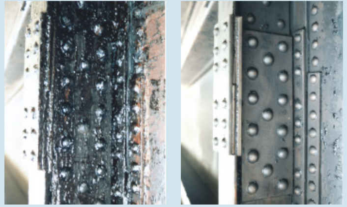
Removing resinated oil for renovation purposes.
